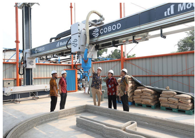
Fig. 1 A fully automated construction machinery 3d printing concrete structures with assured workmanship
