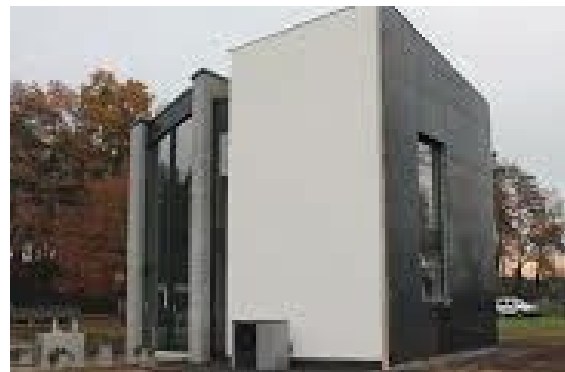
Fig. 6. Two-story 3D-printed house-kamp C
